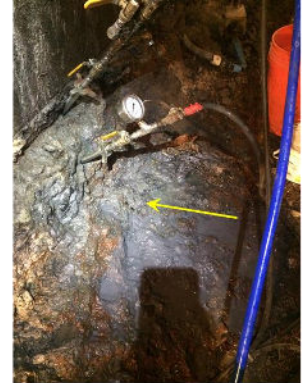
NOH2O Sealing the Leak
