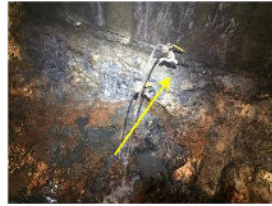
Drilled Hole with Packer
